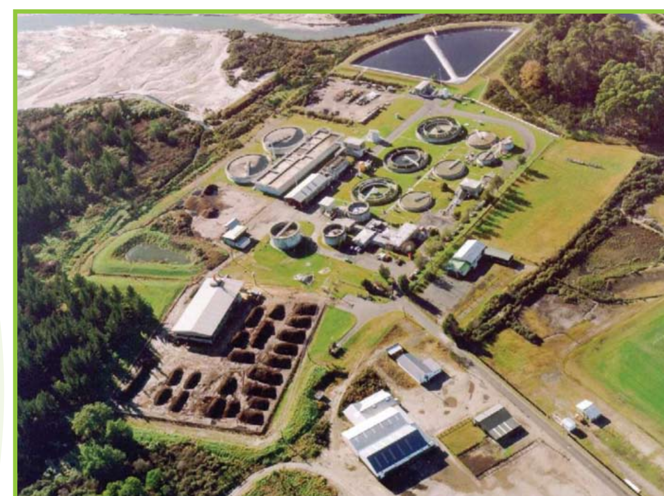
Rotorua Wastewater Treatment Plant
