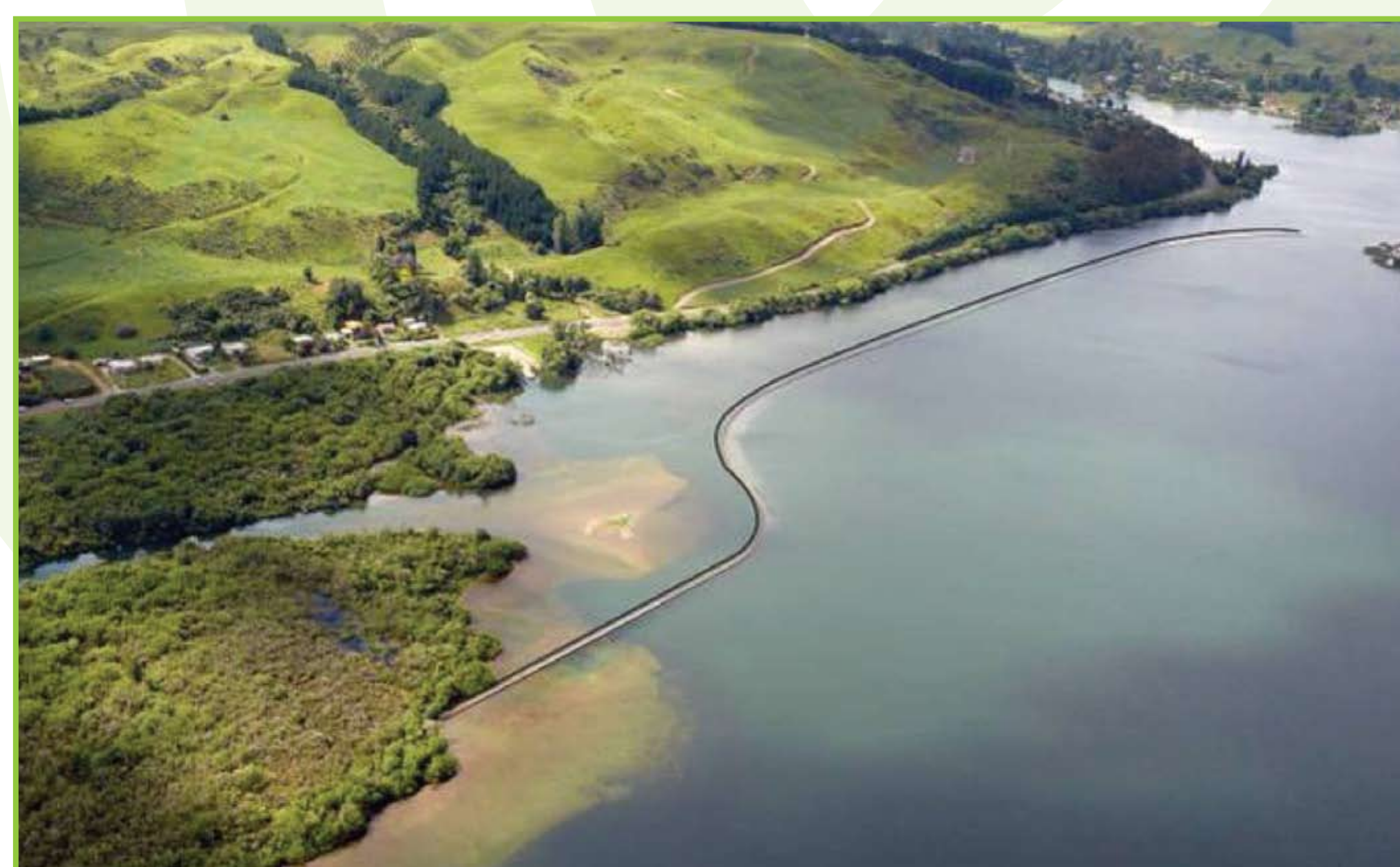
Ohau Channel Diversion Wall
