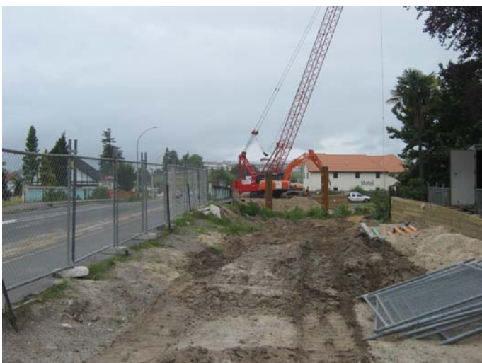
Pile work continues on Utohina Bridge
