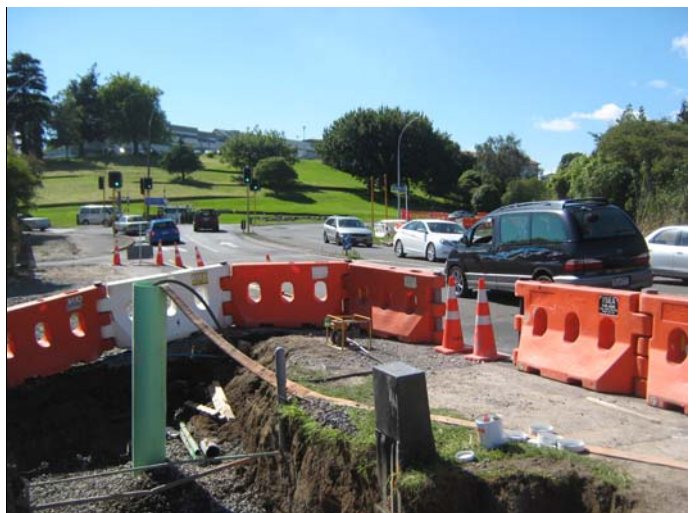
Water is pumped as service cables are pulled through ducts
