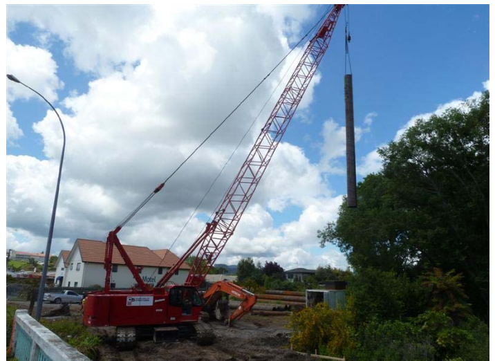
Utuhina Bridge Piling
