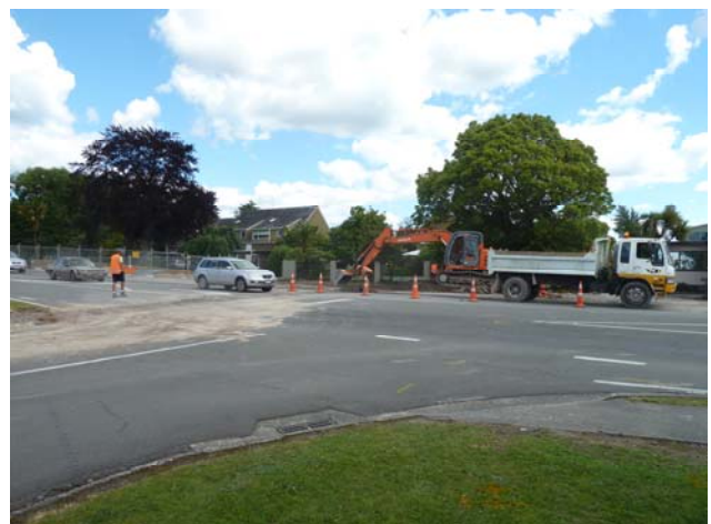
A service trench crossing across Lake Rd
