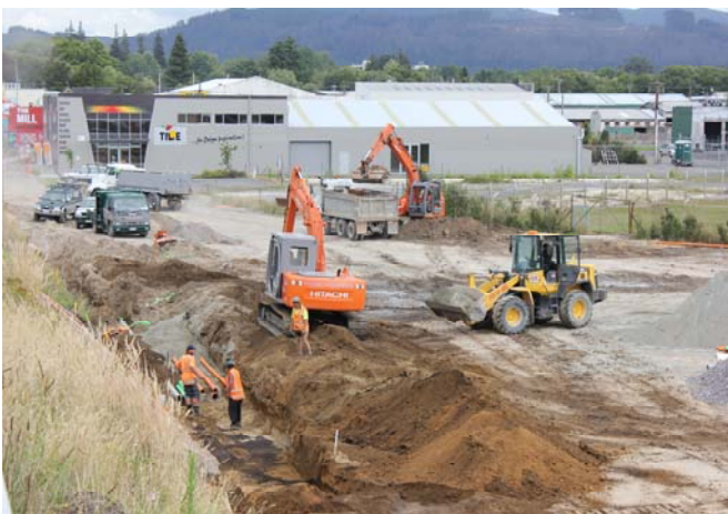
Ducts being laid alongside Railway Bridge
