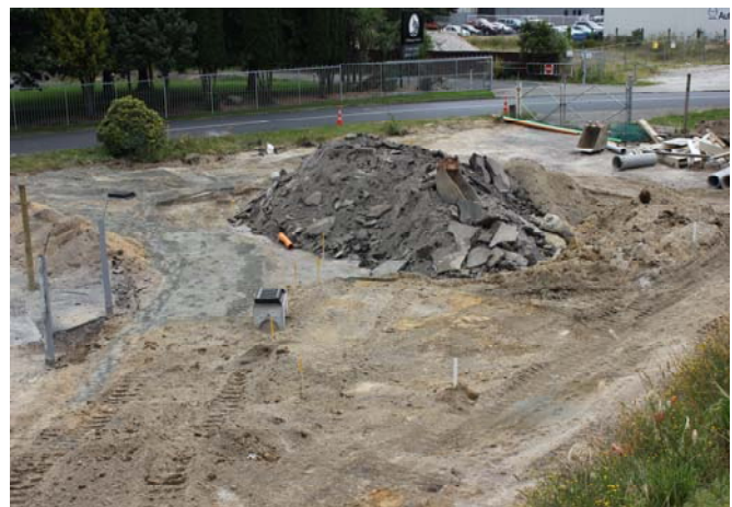
Preparation of the new Dinsdale St entrance
