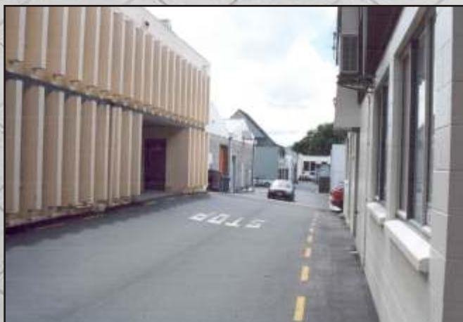
A well used service lane. A total of 248 lots are affected by the service lane requirement and of these, lanes have been acquired from 71 lots or 30% as at December 2002
