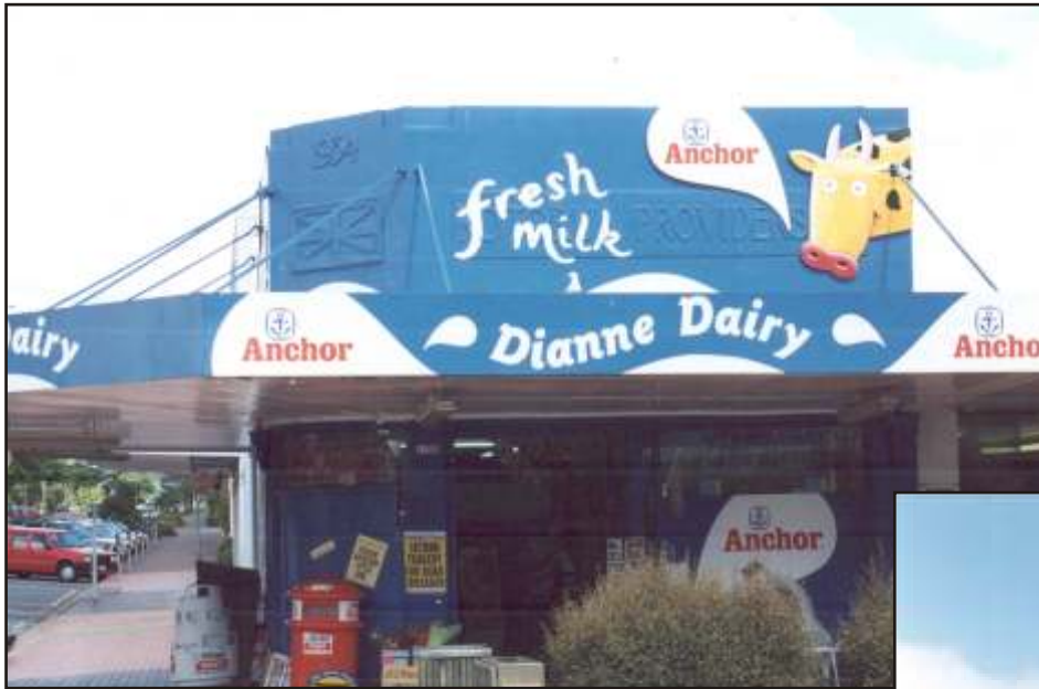
☹ The bright paintwork and advertising obliterates the building's detailing
